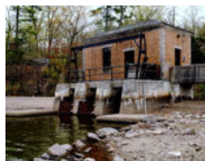
State doing maintenance on Greenwood ...
