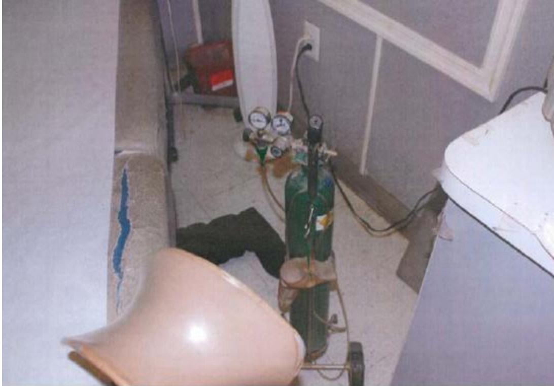
Procedure room, depicting ripped procedure table & stirrup, dust-covered oxygen tank, corroded tubing,
