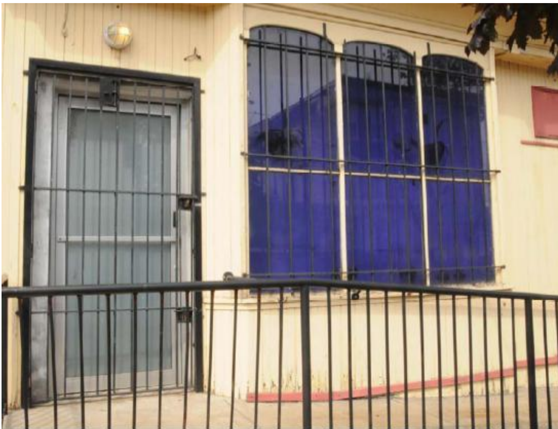
Locked emergency access to Gosnell's clinic
