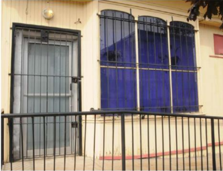
Locked emergency access to Gosnell's clinic
